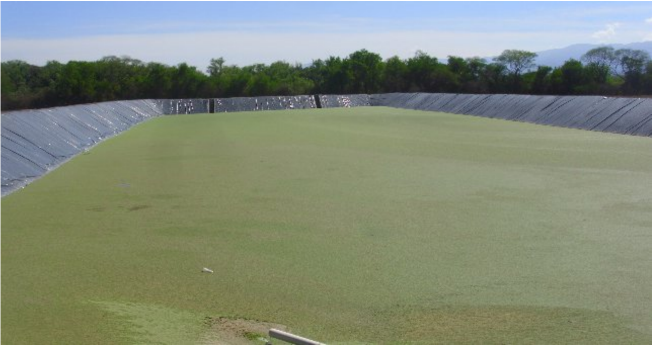
Illustration 2: Small (~1ha) secondary wastewater lagoon at El Carril in Salta, Argentina.
