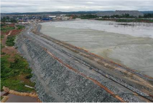
Figure 4: Drone imagery of the southern embankment of the Tailing Storage Facility (TSF) at New Liberty Gold Mine, Liberia
