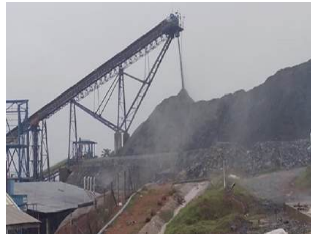
Figure 2: Ore Crushing Plant at New Liberty Gold Mine, Liberia
