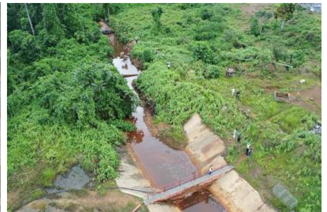
Figure 7: An image of a channel which conveys gold mine effluents from the TSF into the environment
