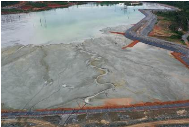
Figure 6: Drone imagery of the western embankment of the Tailing Storage Facility (TSF) at New Liberty Gold Mine, Liberia.
