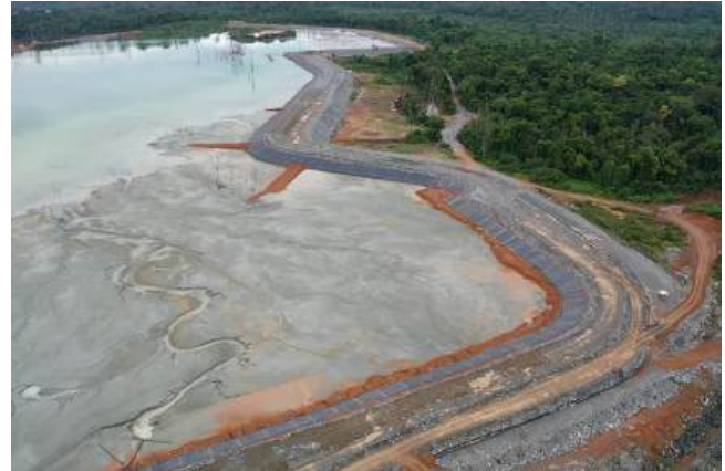
Figure 5: Drone imagery of the northern embankment of the Tailing Storage Facility (TSF) at New Liberty Gold Mine, Liberia.
